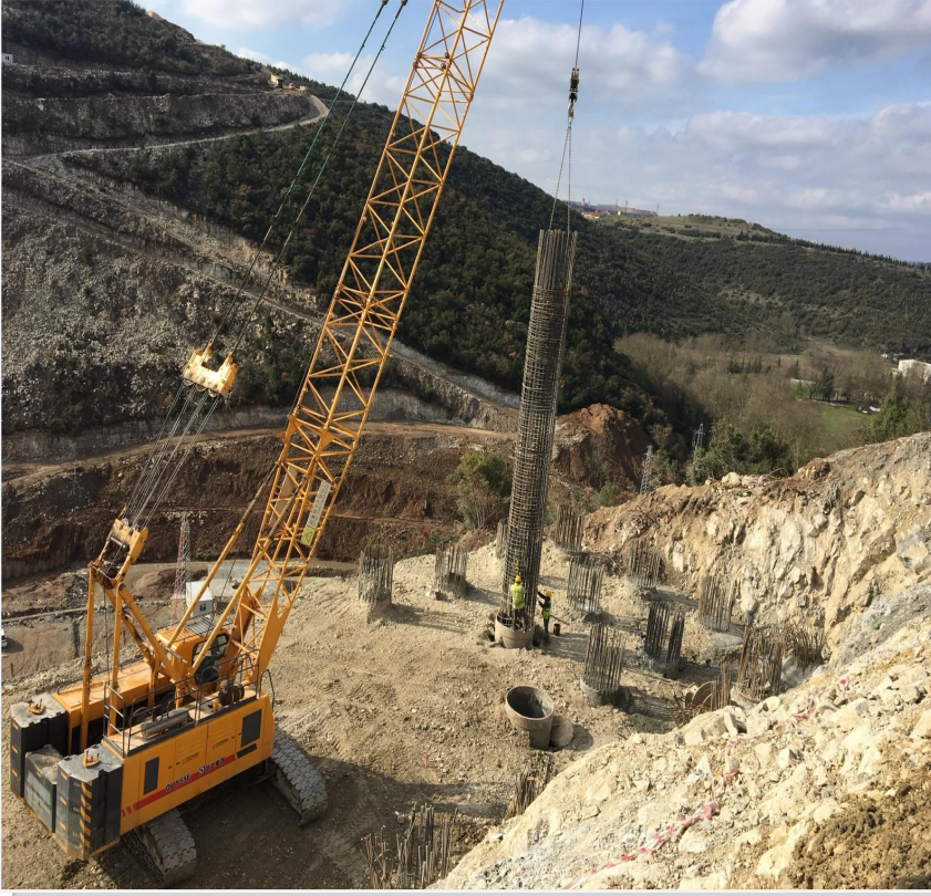
NORTH MARMARA HIGHWAY - DILOVASI
